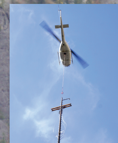
One phase of the repair required a helicopter to carry several thousand pounds of poles and wires. Expert piloting and surgical precision were required to put these assets in place safely.
